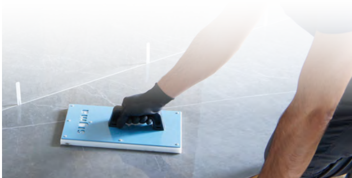
Beat Tile Trowel 16x33 cm, specific for the correct expulsion of air from under the tile.
